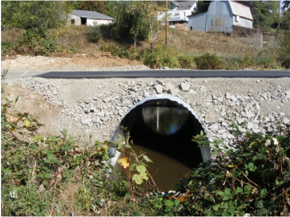
Badger Creek culvert replacement
