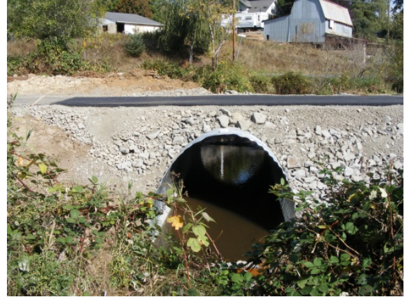
Badger Creek culvert replacement
