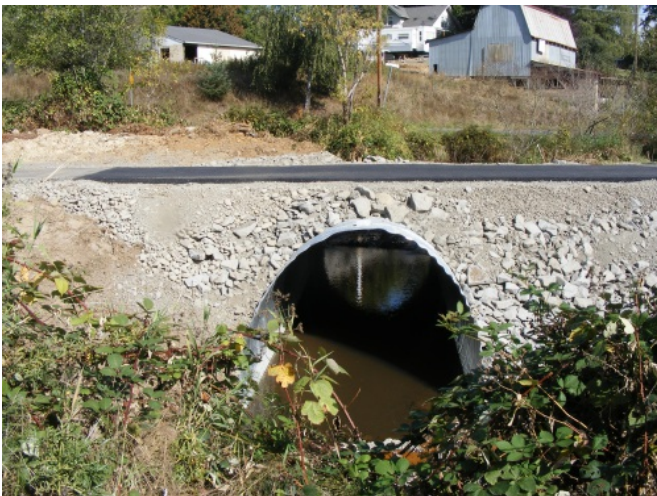
Badger Creek culvert replacement
